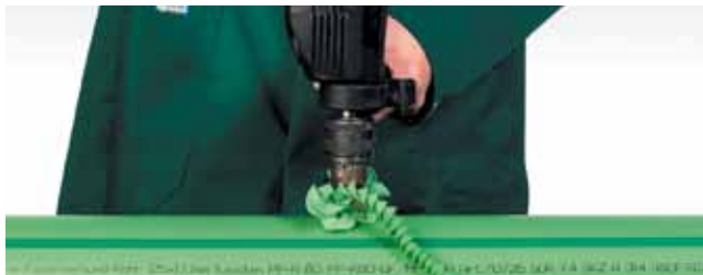
Drilling through the pipe wall
