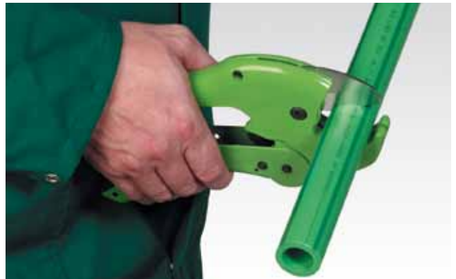
Cutting of the pipe
