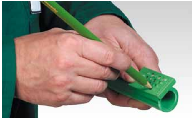
Marking of the welding depth
