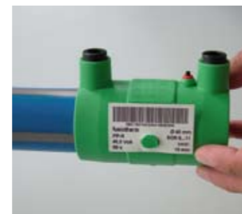
Push the electrofusion socket onto the pipe end
