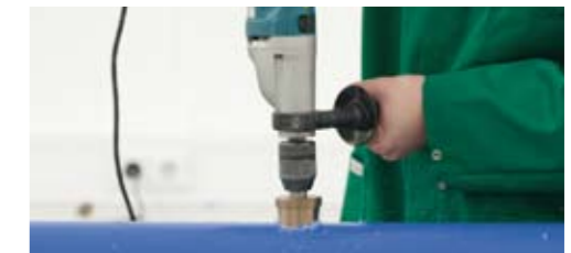
Drilling through the pipe wall
