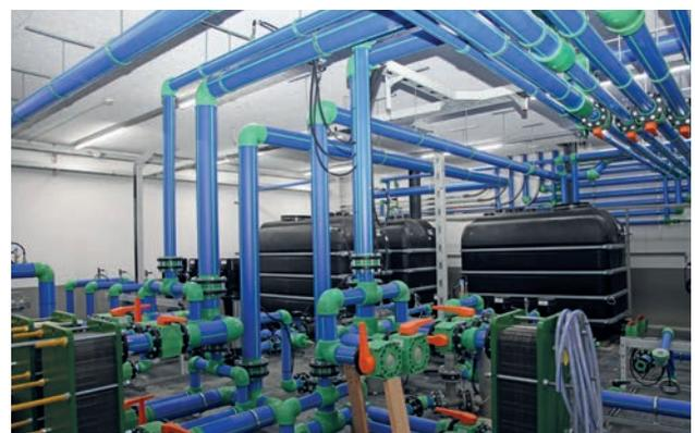
aquatherm blue pipe was installed to provide process water.
