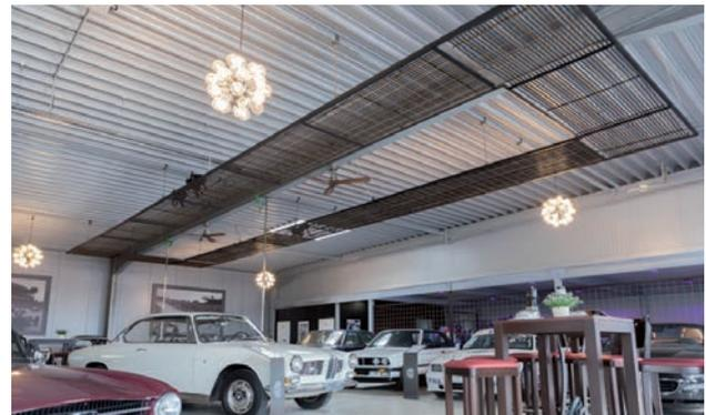
In the showroom of Depot3, the aquatherm black system panels were mounted on a steel frame suspended from the hall ceiling.
