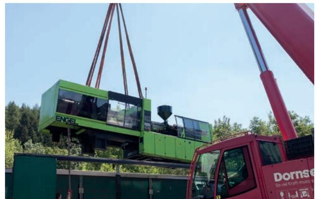
Relocation of injection-molding machines and loading with a crane.
